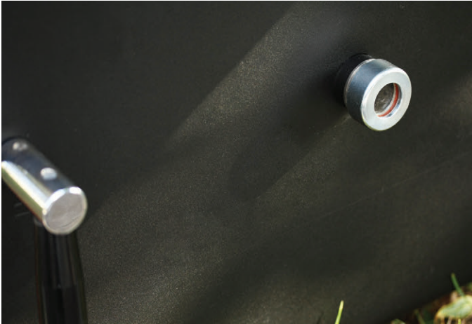
Observation Glass to Monitor Gasification Process
