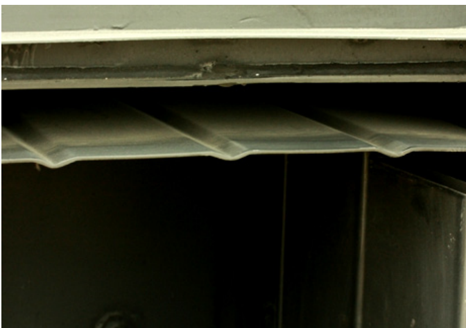
Bypass system automatically engages and prevents smoke bursts when the door is open meeting highest Health and Safety Standards in force.
